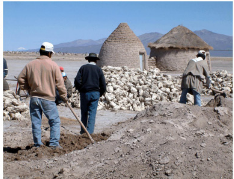
CHIPAYANS CONSTRUCTING A COMMUNITY CENTER
